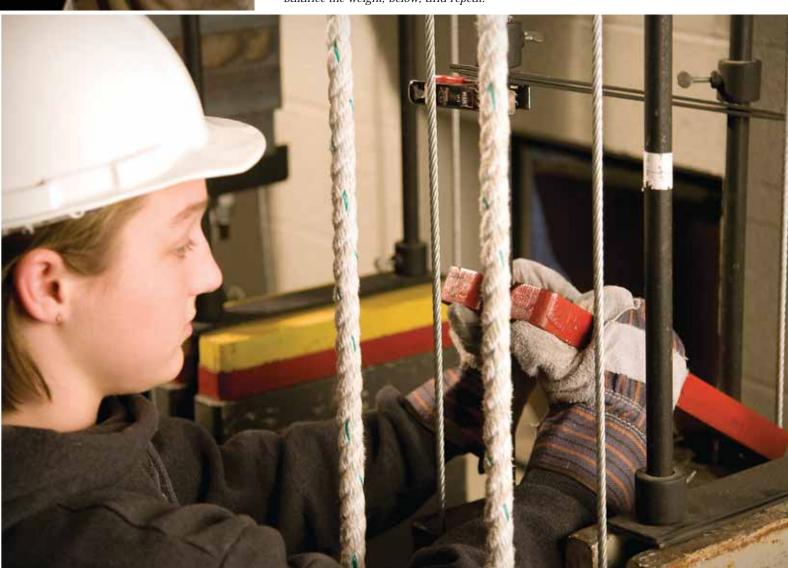
counterweight system, in particular the loading and unloading of counterweight, is more difficult and, if not handled properly, dangerous.
